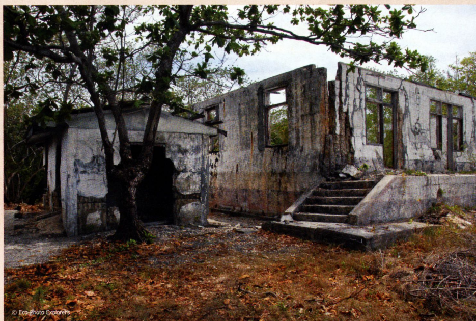
The original keeper's house for the Apo Reef Lighthouse is in ruins. The memories of the lighthouse keepers who lived here have disappeared into the pages of time.
