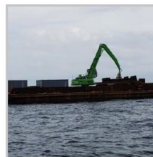
Material from the demolished Tappan Zee Bridge being deposited
